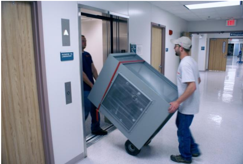
FANWALL® Cell Replacement
